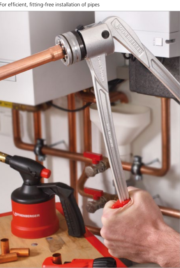
Standard screwable expander head, still compatible with the ROLOCK Expander
